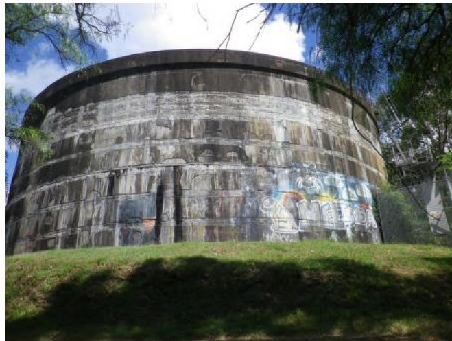
Cessnock Water Supply Reservoir (RPS 2016)
