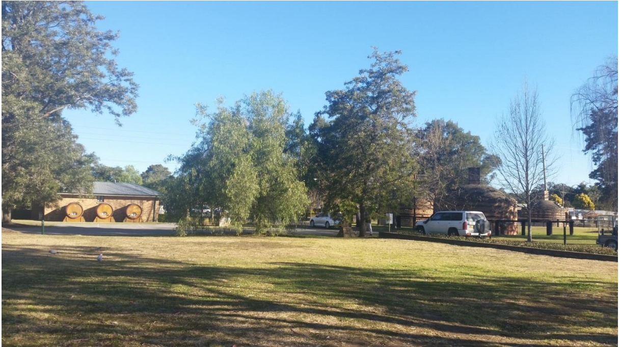
Figure 34: The kilns of historical significance are on the right hand side and the tourist and visitor accommodation is located on the left hand side. The kilns are separated from the tourist accommodation by an access road.
