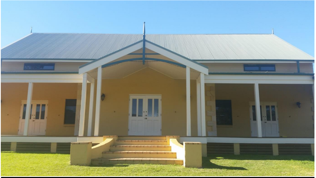
Figure 25: The new Pokolbin Community Hall that replaced the original community hall following a car crash.
