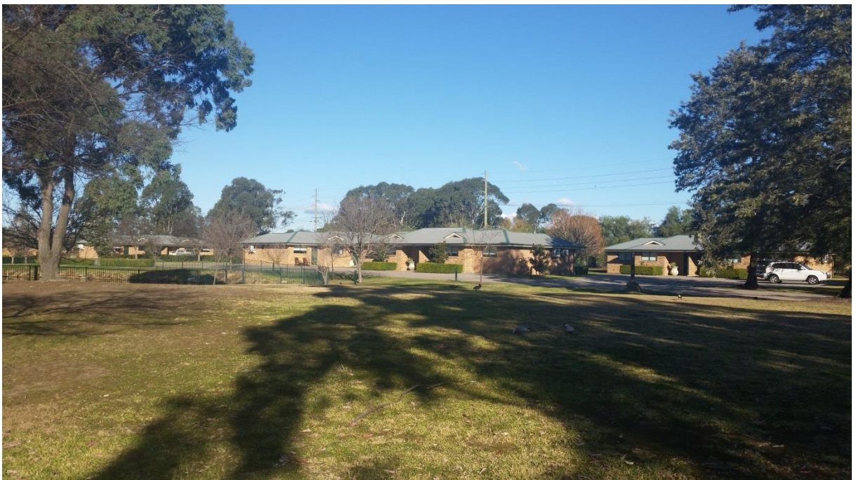
Figure 35: The tourist and visitor accommodation that is now located on a separate lot to the kilns that are of historical significance.
