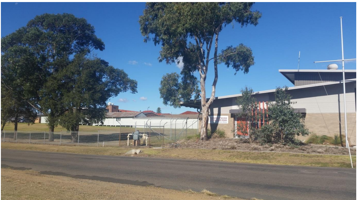
Figure 31: The Cessnock Hospital Buildings (dark red roof) can be seen in the distance from the new ambulance station.
